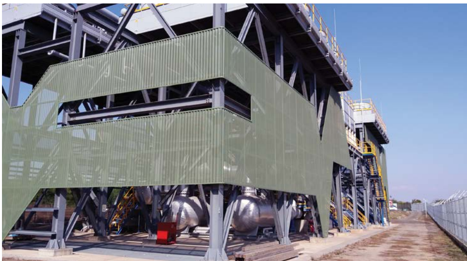
The first geothermic power-plant in Hungary, Tura
