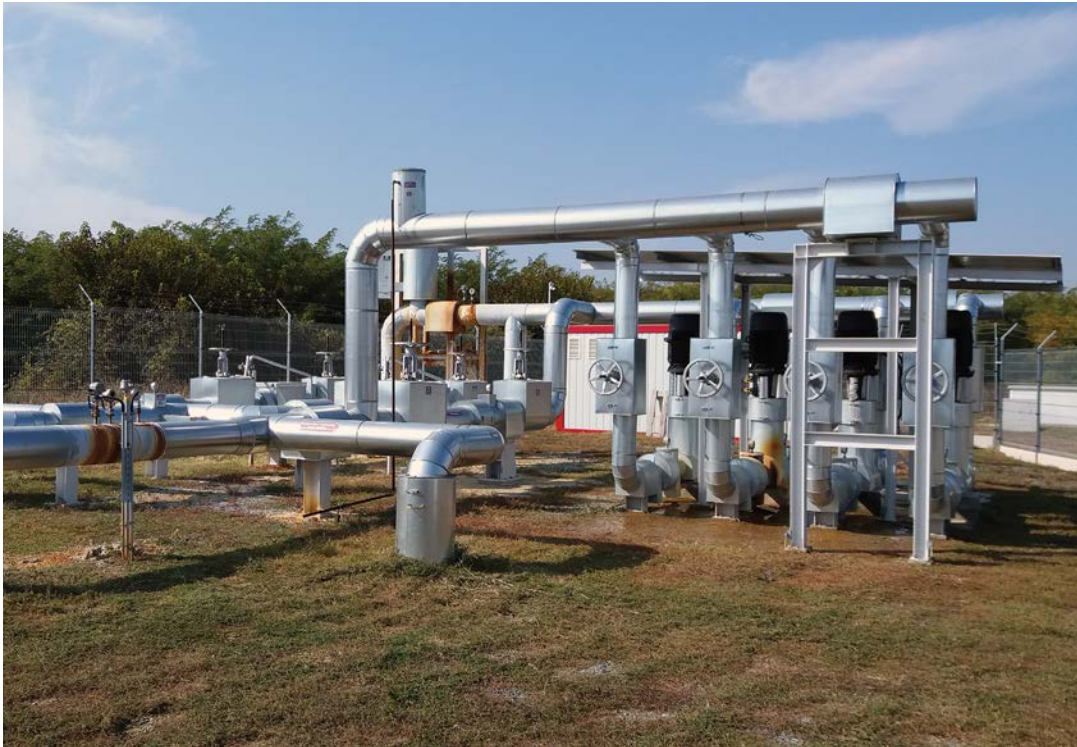
Thermal water injection well in Tura
